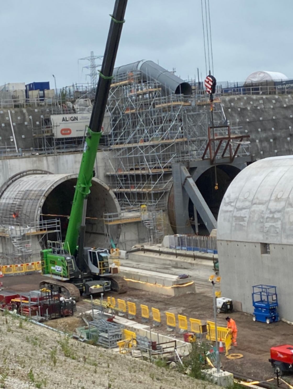
The Railway group visited the HS2 construction site at Maple Cross and had a guided tour in a minibus. Picture: Jane Campbell
